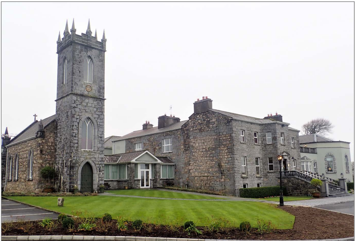
Illus. 10—The house and its chapel are now part of a much larger building group, within landscaped grounds with golf course, forming the Glenlo Abbey Hotel
