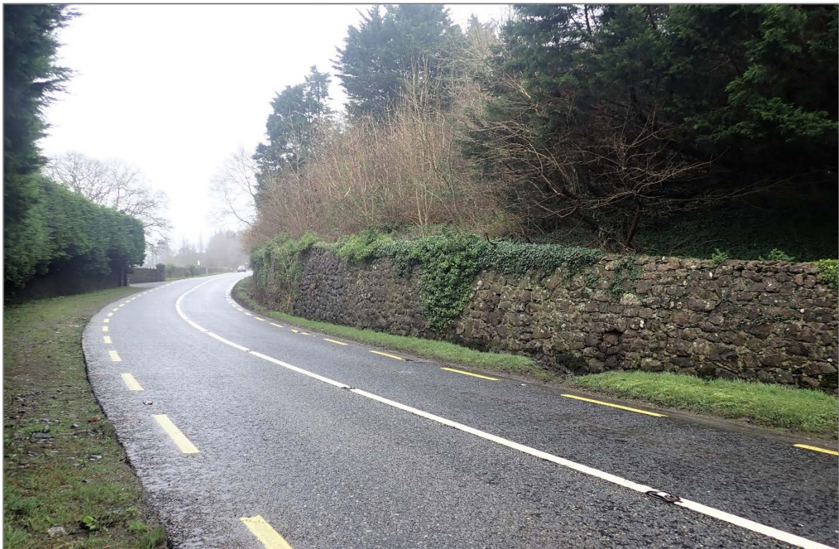
Illus. 15—Looking east along the N59 showing a substantial wall in mortared granite rubble, which seems to be a remnant boundary wall of former Riverview House.
