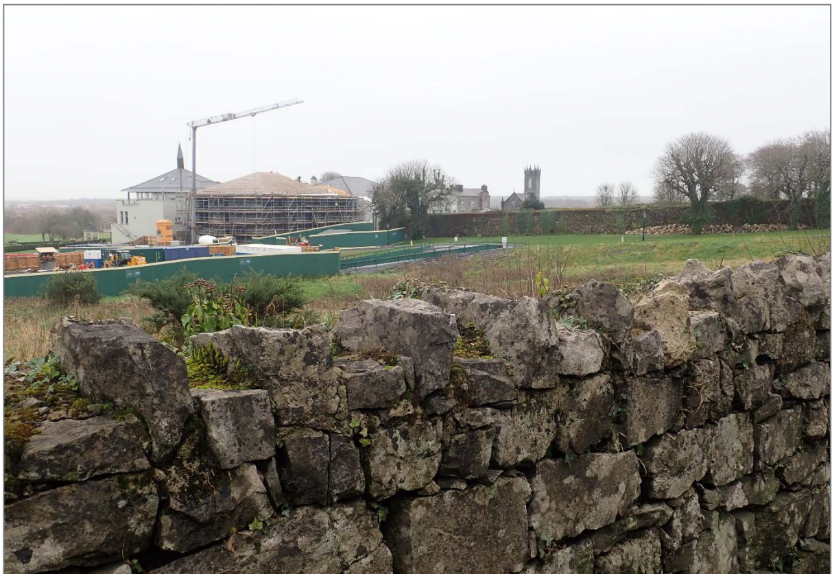
Illus. 12—Towards the west end the roadside boundary of the Glenlo Abbey Hotel is roughly squared limestone rubble with crenelated top course.
